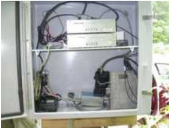
Figure 3 —The vehicle and bicycle counters shared a single radio that transmitted their data.
